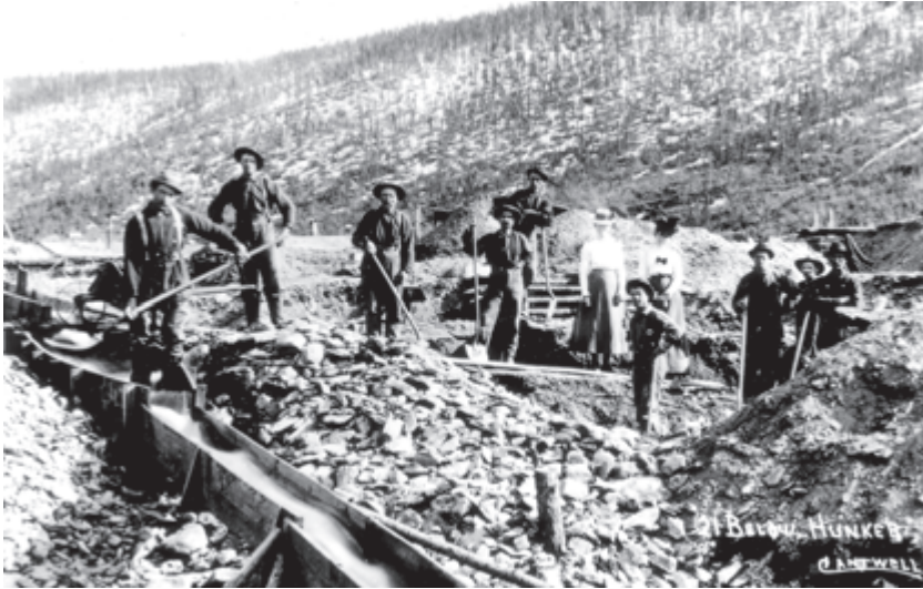
Fig. 9. Early summer on the creeks, with a group of miners shovelling into their timber sluice the ore and debris from a winter's underground digging. The photographer's inscription refers to the twenty-first claim downstream of the first claim on Hunker Creek (photo: Turnbull Collection, Dawson City Museum).
