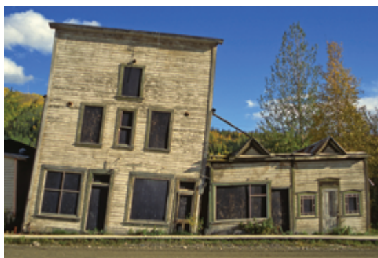
Fig. 15. Old houses in Dawson, subsided over thawed permafrost.
